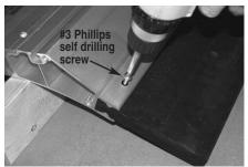
b) Using Phillips #3 bit, run a self drilling screw into each of the four pilot holes. This prevents rubber from movement.
